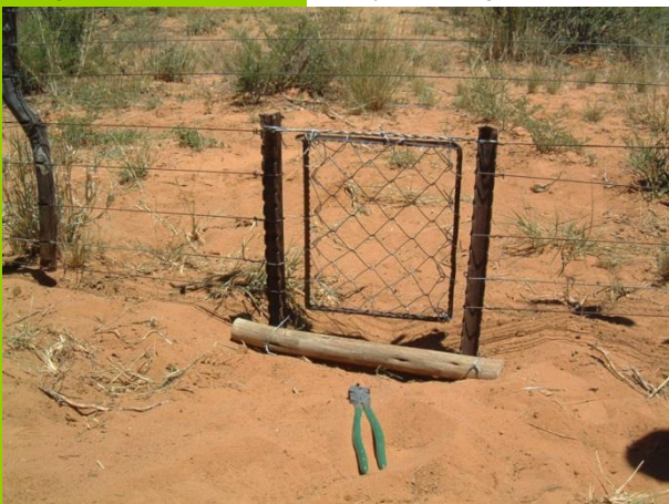
The design of the swing gates in a game fence. Swing gates are similar in concept to a residential pet door. They enable burrowing animals such as warthog, cape porcupine and aardvark to enter farms through a hinged flap in the fence line.
